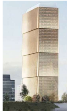
Timber Marina Tower
